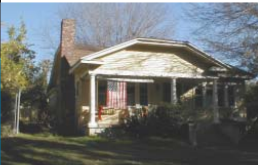
This cottage has been preserved by retaining its clapboard siding and wood windows.
